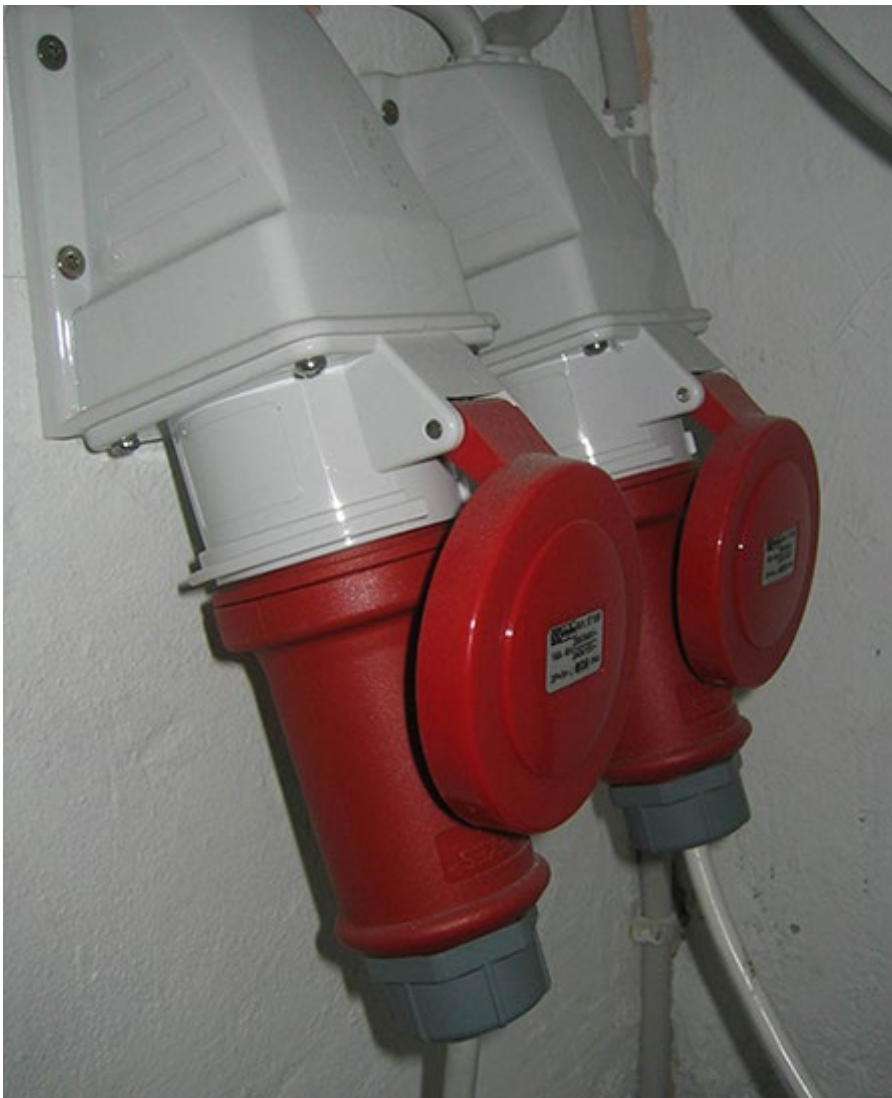
Figure 5: This red color-coded heavy-duty connector satisfies the IEC 60309 standard for supplying 380 to 480 V. (Image source: Wikimedia Commons )
