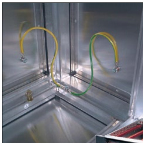
Earthing of removeable parts in a cabinet
