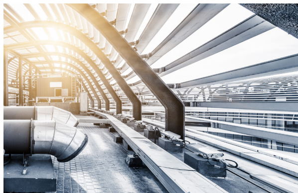
The G120X can be operated with any motor, but most effectively with synchronous-reluctance motors from Siemens.
