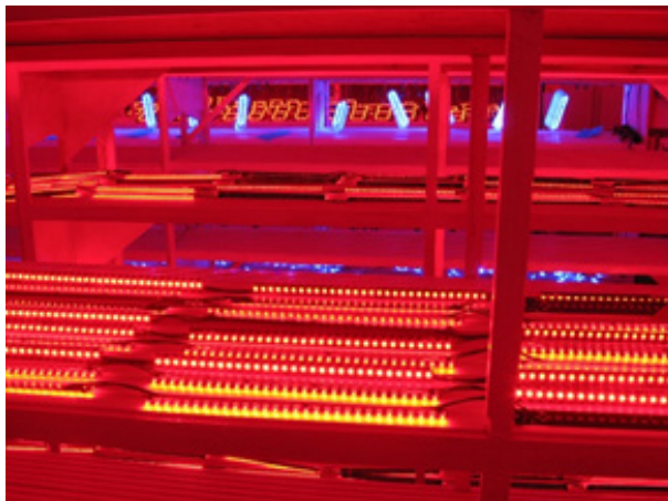
Burn In of flexible strip displays used for auto gas station pricing signage
